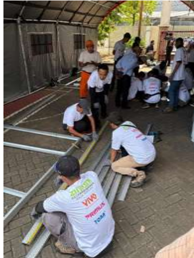
Figure 6. Light Steel Construction Installation Practices
