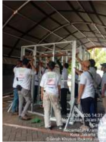
Figure 8. Prototype of Light Steel Ceiling and Partition
